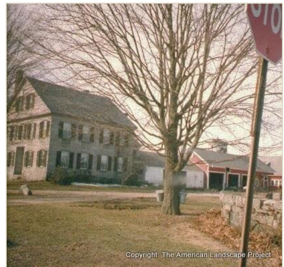
Figure 2-2: Temple Front House with attached barns, Keene, NH. This house features a series of attached barns. Consider the dangers and benefits of this design strategy. Note the sap buckets hanging from the tree in the foreground.
